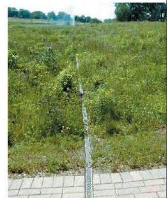
filter strips/level spreader
