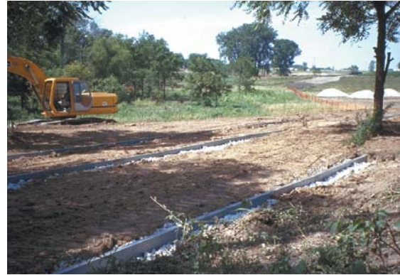
Coffee Creek Center level spreader installation (Chesterton, IN) (Conservation Design Forum)
