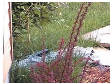
roof down spout connects to rainwater garden (Glen Ellen, IL)
