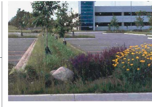
bioswale in a parking lot (Tellabs, Naperville, IL) (Conservation Design Forum)
