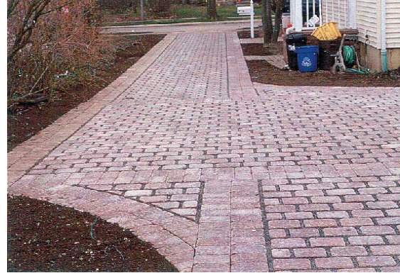
porous pavement driveway
