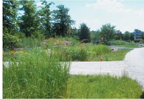
vegetated swales planted with native grasses and forbs along the street
