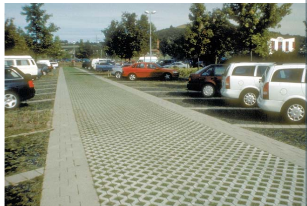
porous pavement in parking lot
