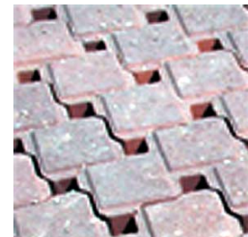
porous pavement allows infiltration through the paving material
