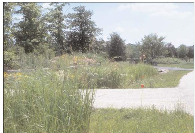
Swales with native plantings retain and cleanse stormwater runoff. Narrow lanes reduce pavement area and travel speed.
