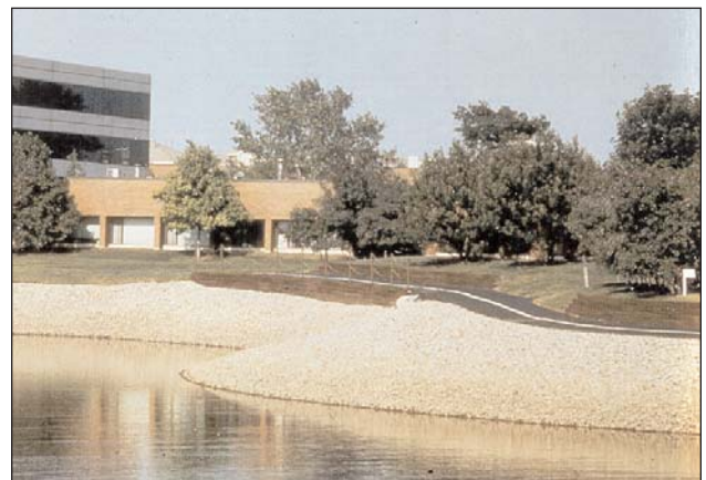
Detention ponds with rip rap edges provide no water quality benefits and have limited aesthetic quality.
