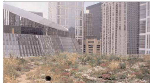
Chicago City Hall green roof insulates the building, provides wildlife habitat, and reduces roof runoff.
