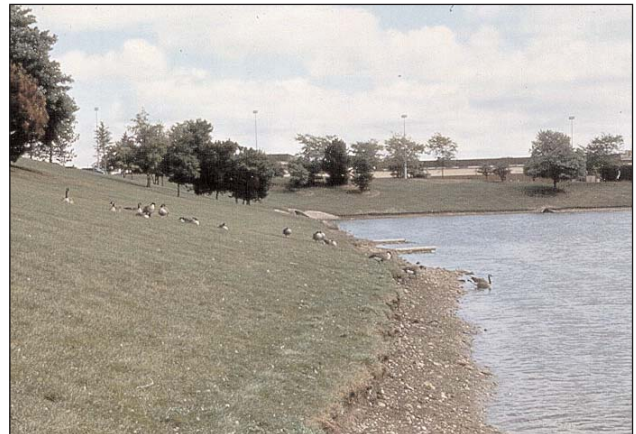
Turf lined stormwater detention typical of conventional development leads to shoreline erosion and supports excessive goose populations that cause water quality problems and reduces recreational use.
