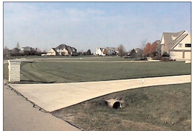
Although producing less runoff than curb and gutter systems, turf swales subject to wet conditions may lead to bare ground and subsequent erosion as well as reduced aesthetics.
