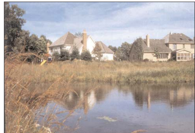
Naturalized detention provides desirable stormwater treatment and wildlife habitat while discouraging geese and enhancing rural character.
