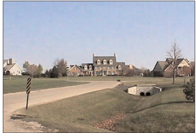
Turf grass stormwater drainage systems often lead to dead grass and bare ground due to wet conditions and subsequent erosion.
