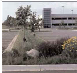
Parking lot with bioswale to filter and absorb runoff. Shade trees reduce heat gain.
