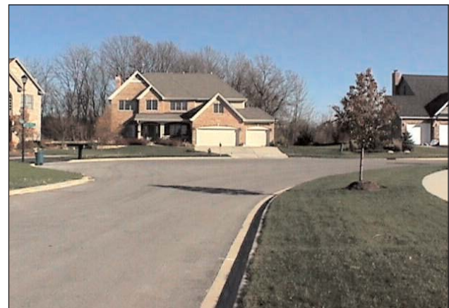
Large setbacks increase total pavement and imperviousness. Street “eyebrows” and curb radii increase impervious surface area and encourage inappropriately high automobile speeds.
