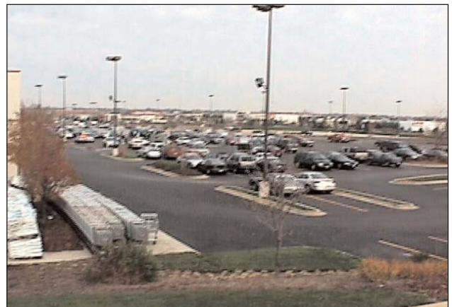
Conventional commercial sites have a high percentage of impervious surface, and can require significant amounts of storm sewer and detention.
