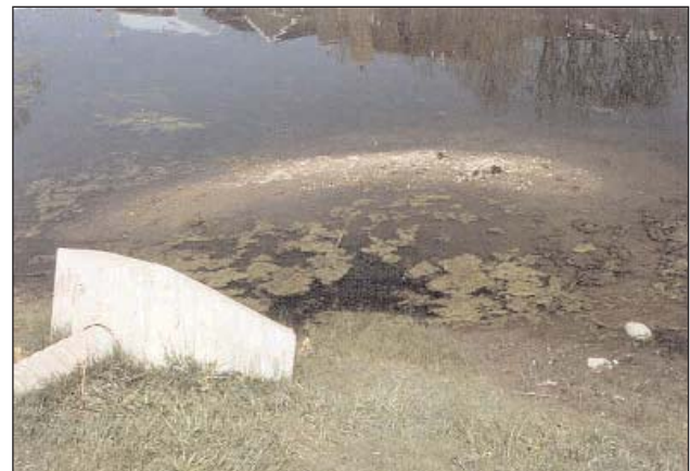
Direct discharge into conventional wetlands is typical. Heated and untreated stormwater can disrupt the natural ecology of a wetland.
