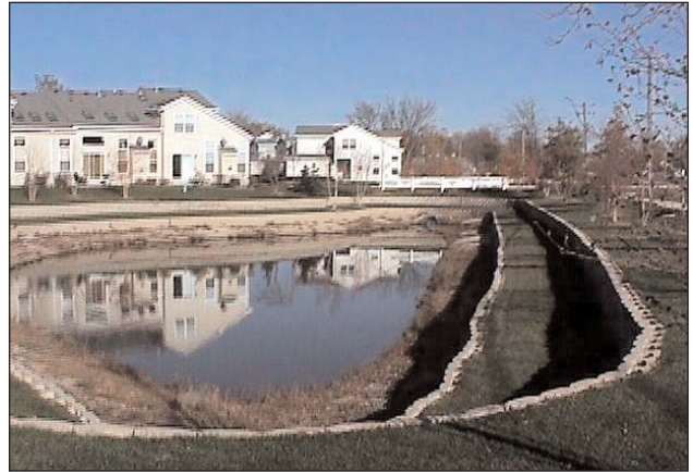
Reliance on conventional detention as a sole stormwater management technique leads to unaesthetic conditions and decreases quality of life.
