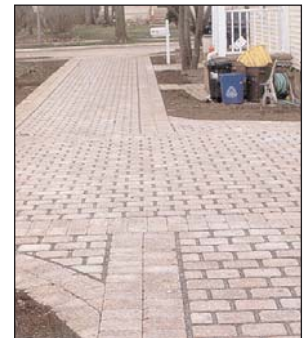
Conservation residential developments may use porous pavers for driveways and off-street parking areas. (However, the evaluation modeling assumed no porous paving.)
