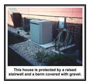
**Precautions:** The berm can only be built so high. It can be overtopped by a flood higher than expected. Being made of earth, it is susceptible to erosion from rain and floodwaters if not properly sloped and covered with grass and maintained. A berm can settle over time, lowering its protection level. The small floodwalls can crack and lose their watertight seals.
