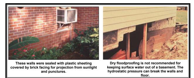
**Precautions:** It is very tempting for the owner of a dry floodproofed building to try to keep the flood out if floodwaters get deeper than two or three feet. This can result in collapsed walls, buckled floors, and danger to the occupants.
