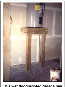
This wet floodproofed garage has bare concrete, unfinished drywall (for fire protection), and an elevated water heater.
